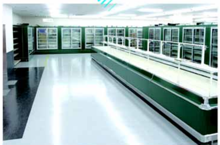
Reach-in type freezing showcase with harmonic oscillating function (Adopted by Okay Store)
